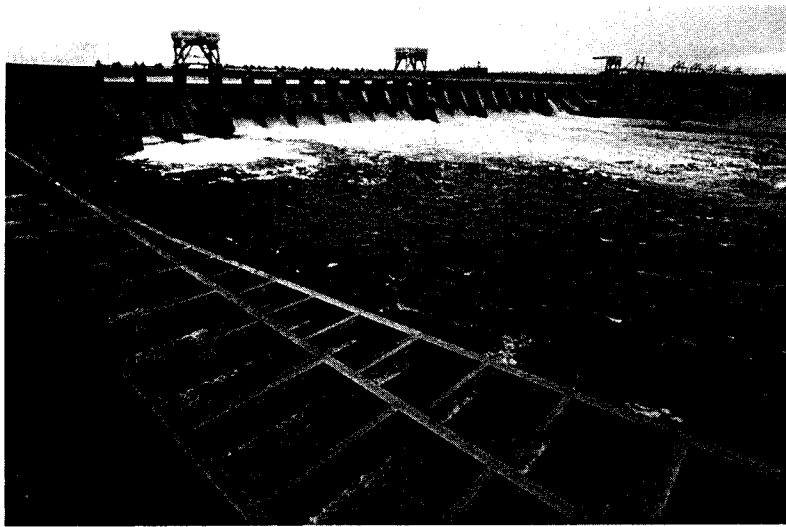
Fish ladders help salmon bypass a dam on the Columbia River. (Courtesy of Bonneville Power Administration Archives)
